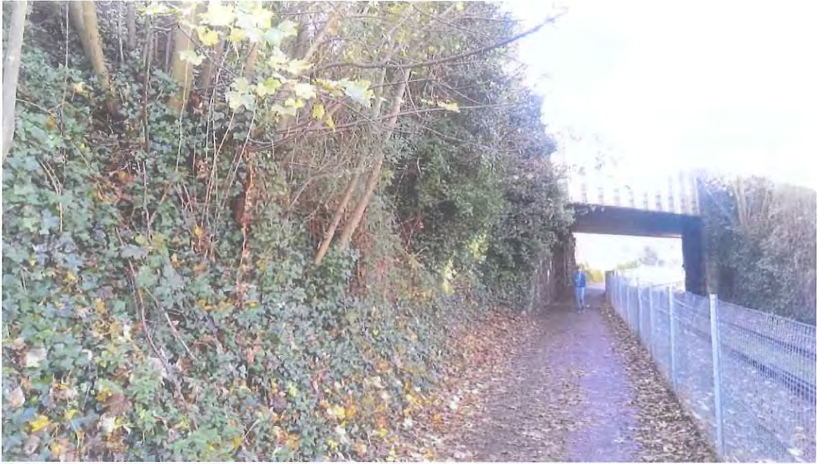
Path from Harbourside to Chocolate Path with Cumberland Road bridge over. Ramps/retaining structures continue under bridge.
