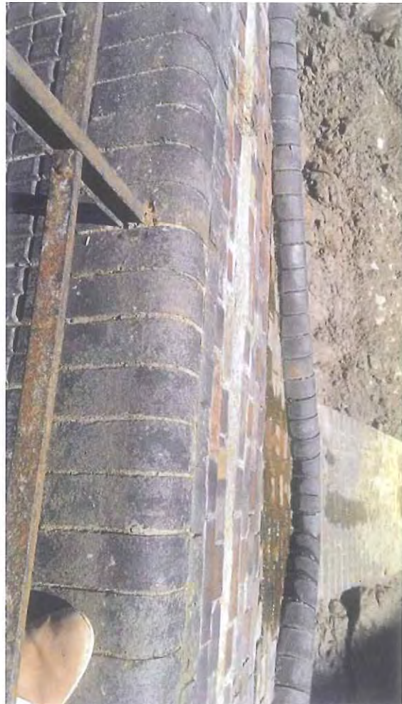
Example of other patchwork along chocolate path and facing materials to retaining wall of river bank (pennant stone with blue bullnose brick capping)
