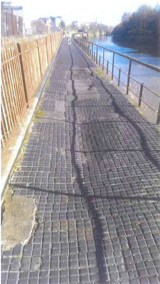
Example of other patchwork along chocolate path and facing materials to retaining wall of river bank (pennant stone with blue bullnose brick capping)
