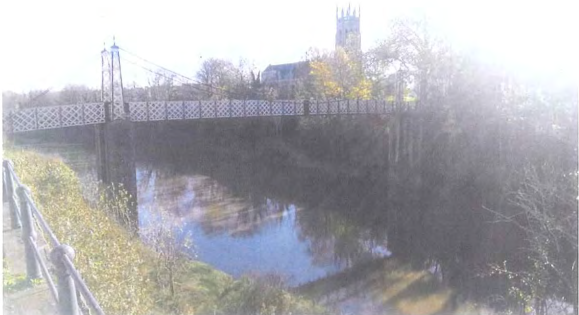
Existing bridge to east - Gaol Ferry Bridge.
